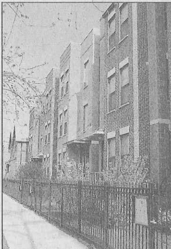
The $17 million Harold Washington United Cooperative consists of 87 units in 18 buildings on 30 lots in the West Humboldt Park neighborhood.
